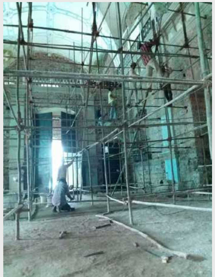
Restoration work in progress at Penha de Franca
