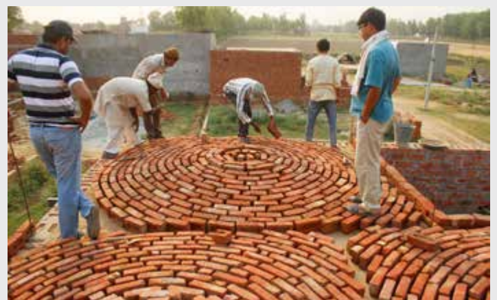
Construction of flat domes in Aryapuri
