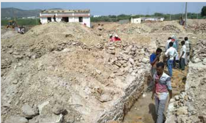
Foundation work in progress at GIDC-1
