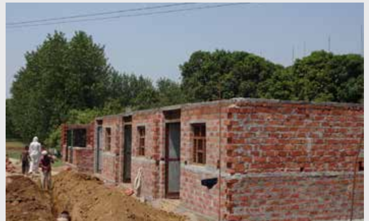
Construction of Houses in Kandhla
